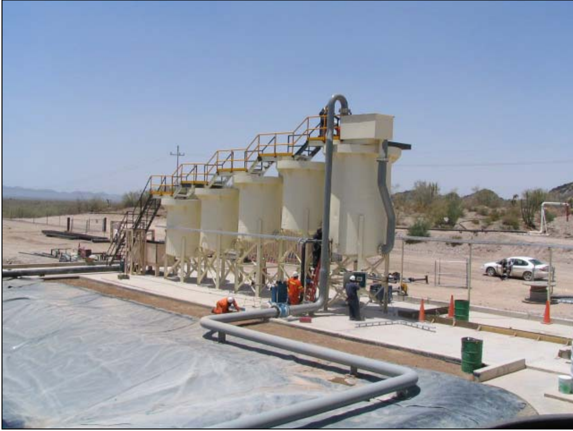
Image 1: New ADR plant construction.
